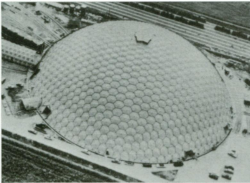
Fig. 6. A steel geodesic dome in Baton Rouge, Louisiana, 117 m in diameter, 35 m high
